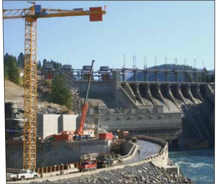
The upgrade of the Waneta Dam is wrapping up.
