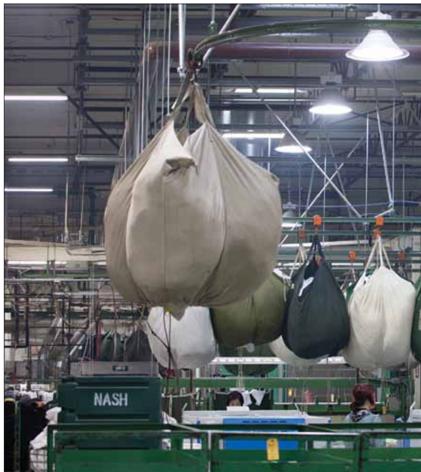
A newly installed overhead transport system allows Teamster member
