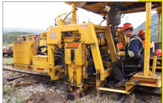
Monte Halladay and Mark Christy (four years with the railway) operate the spiker.
