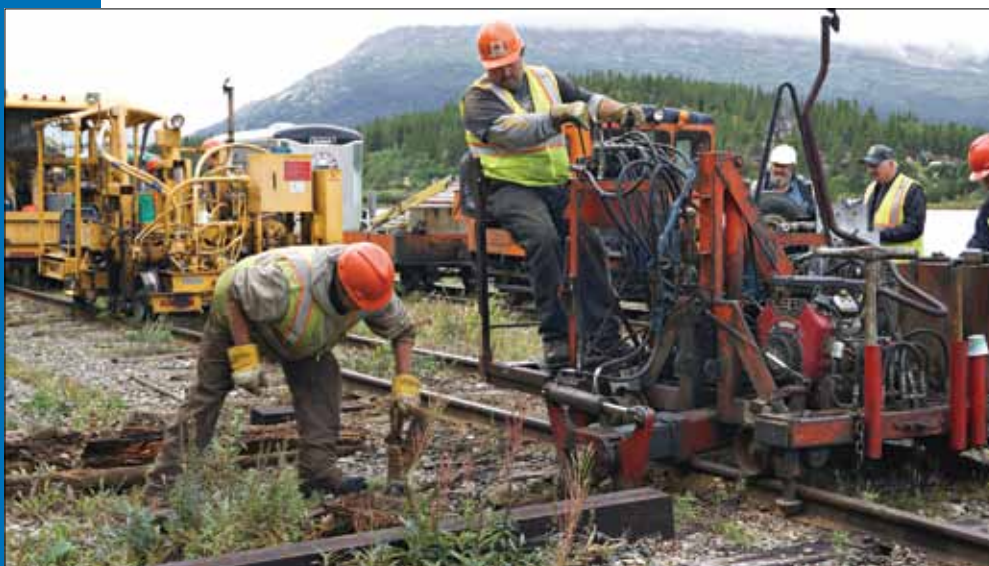
Dale Neumann operates the tie extractor while Andrew James removes chunks of the old railroad ties.
