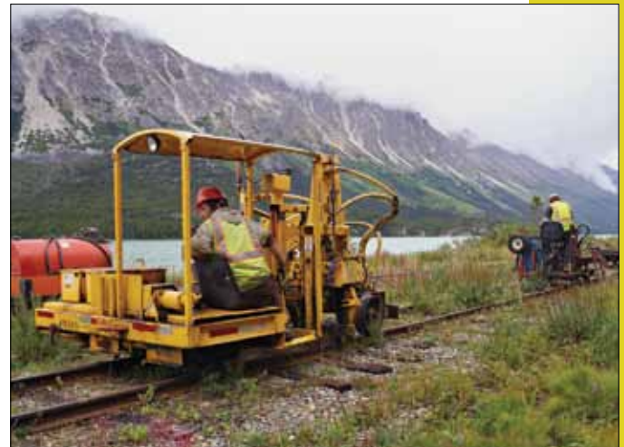
Andrew James and Dale Neumann move track machinery along the siding at Bennett Station.
