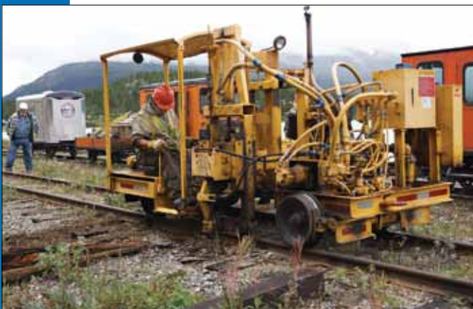
James operates the spike puller with foreman Rick Halladay (18 years) in the background.
