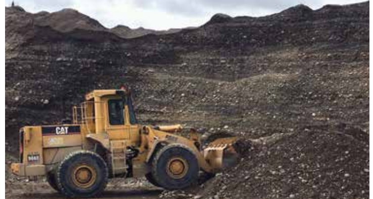
Steve Foisey, operating a loader on a job site in Northeastern B.C.
