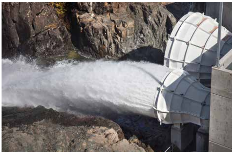
On the downstream side of the dam, the new water release valve directs water down the Elk Falls Canyon.
