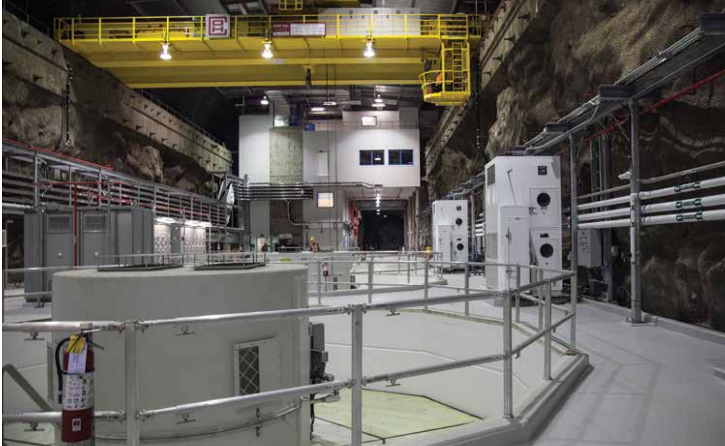
The main floor of the powerhouse showing the location of the three generators with the tunnel in the background.
