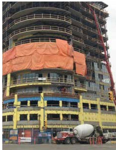
Teamster member Ron Suchocki at OK Ready Mix doing the final pour for Ellis Parc, a 14-storey, 91-unit mixed use high rise adjacent to Prospera Place, in Kelowna.
