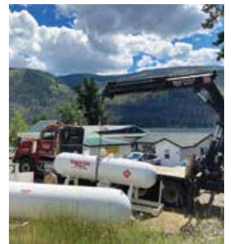
Michael Batchelor is a Teamsters Local 213 member working with Superior Propane at the Marigold Resort at Loon Lake. A propane tank is being swapped out for a new one as per B51 new federal guidelines requiring tanks older than 25 years be replaced with new tanks. He has 40 years in the propane business and is a 16-year member at Superior Propane.
