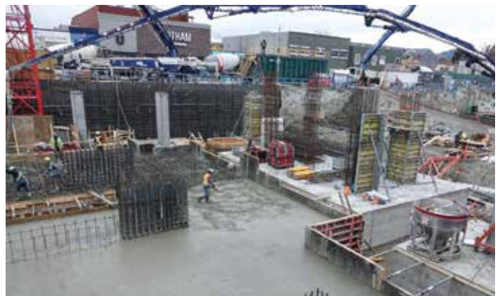
Teamsters Local 213 members pouring approximately 1500m³ of concrete at Water Street by the Park Condo project in Kelowna.
