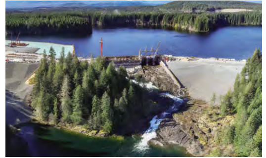
The John Hart Dam upgrade continues in Campbell River.
